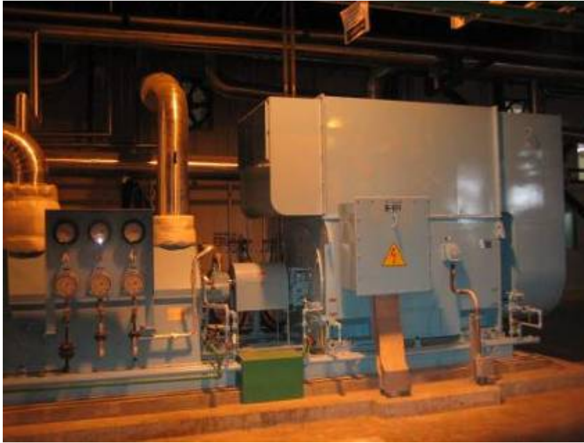
1,450kW 2P 6kV 60Hz TEAAC Motor for Boiler Feed Pump Application at Power Plant
